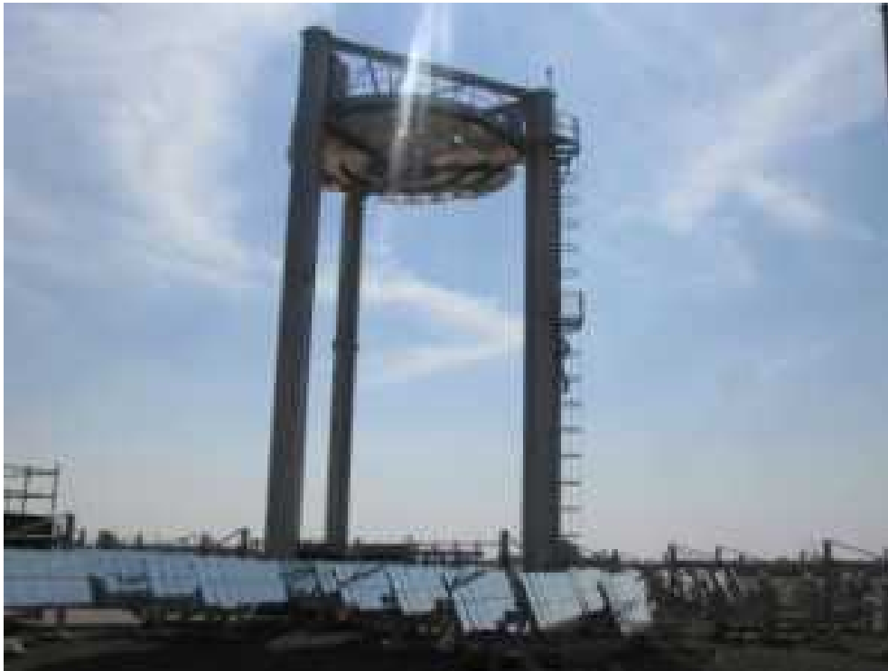
Fig. 12: Beam down solar concentrator (Cassedy, 2000).
